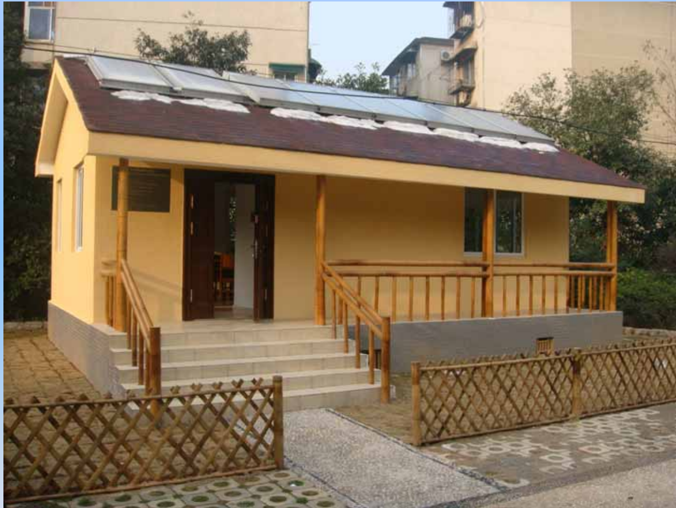
Solar energy/round bamboo demonstration house developed by ICBR and CAF in China
